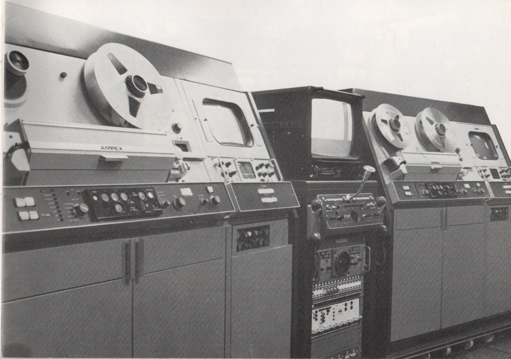
Video Tape-recording Machines in a Transmission Suite. The central console holds monitoring and test equipment
