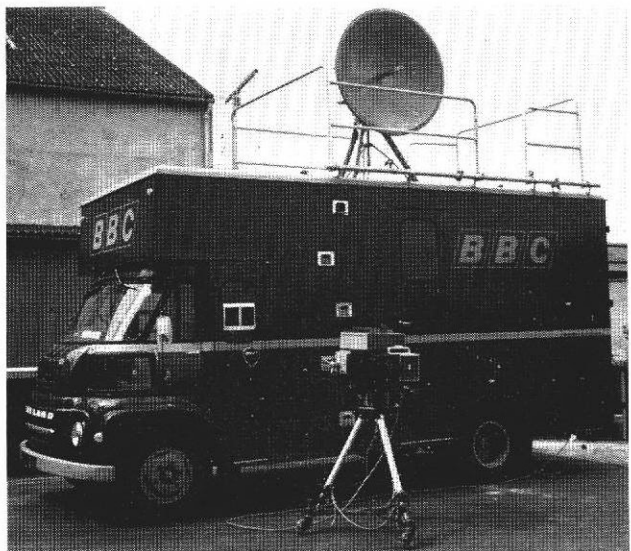
Fig. 3 Two-channel news colour OB unit with Marconi Mk VIII camera
